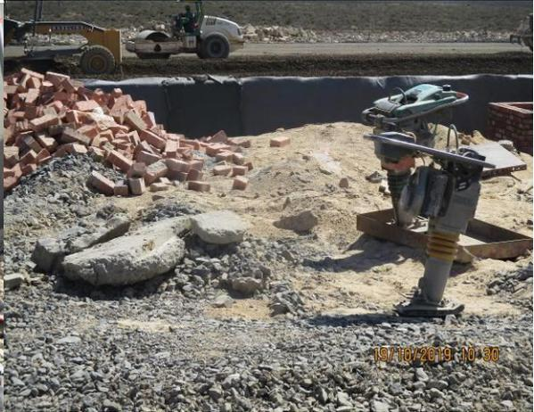
Photos: Small plant place on the ground without drip tray.
