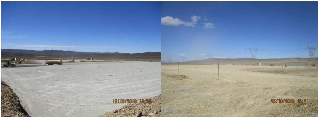
Photo: Final layer at section C.
