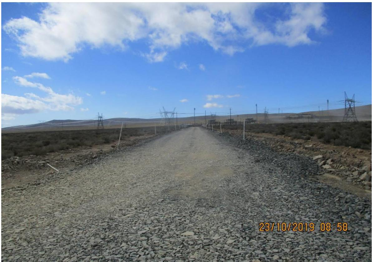
Photo: Layer works on permanent access road.
