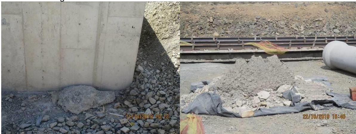
Photos: Unattended concrete waste (not properly cleaned or disposed).
