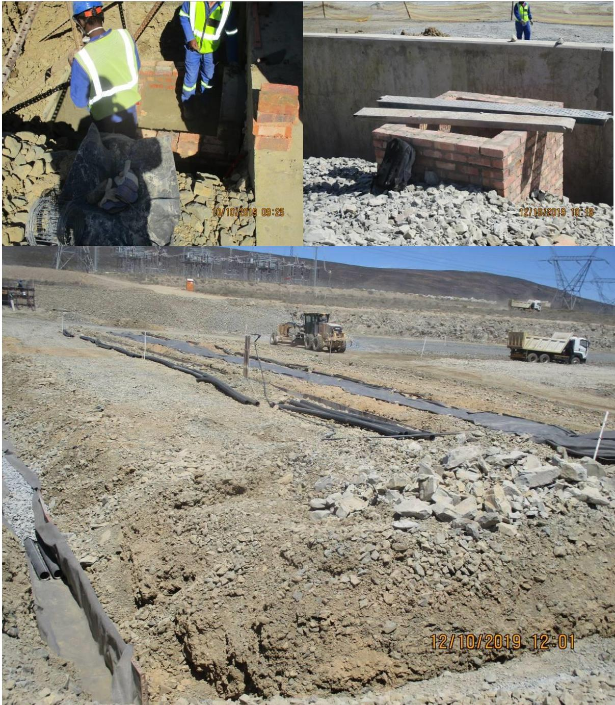
Photo: subsoil drainage mine hall in progress.
