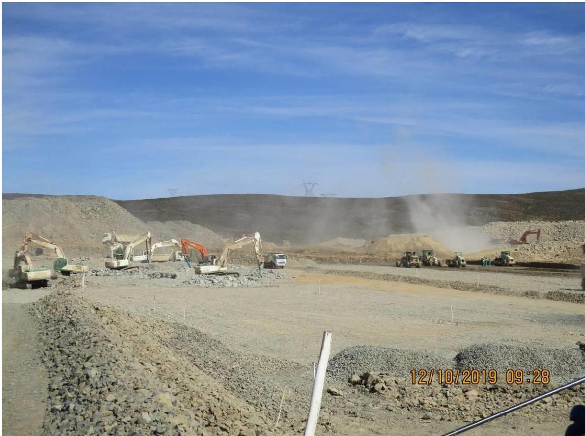
Photo: Breaking of rocks and layers works at section D 400kV terrace.
